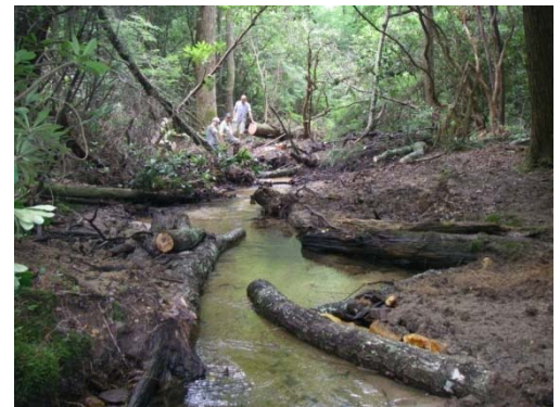
Figure 2 – In-stream structures, such as these deflectors, are built with natural materials that reduce degradation of the stream environment and improve trout habitat.
